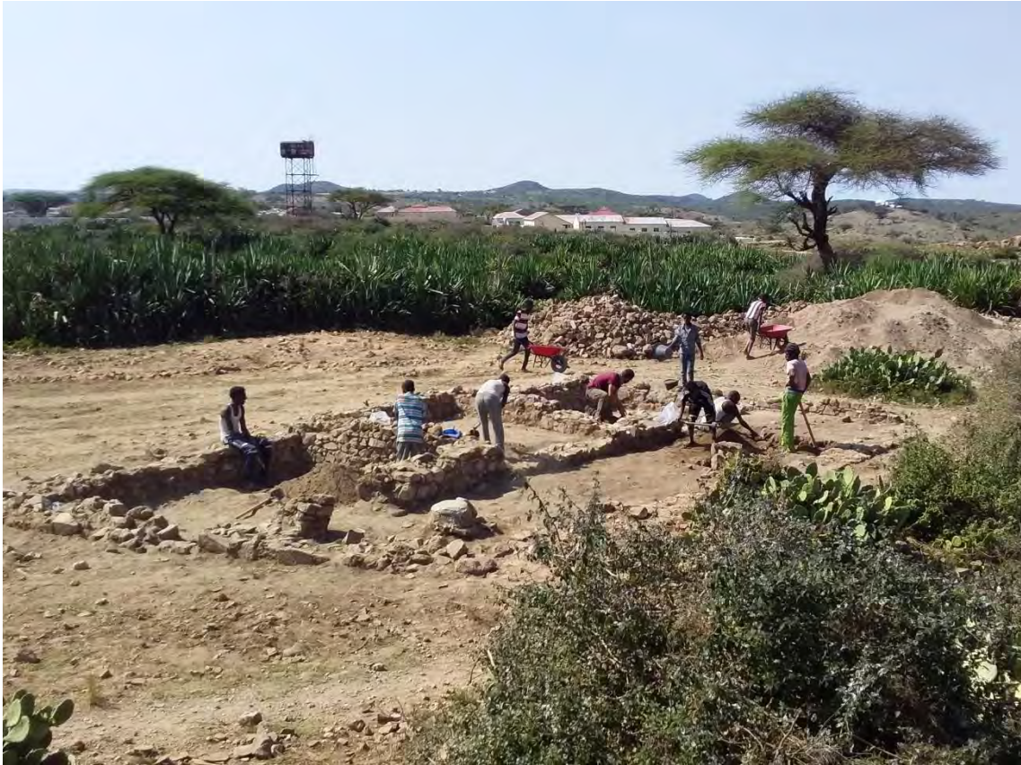
Excavation process of C-3000
