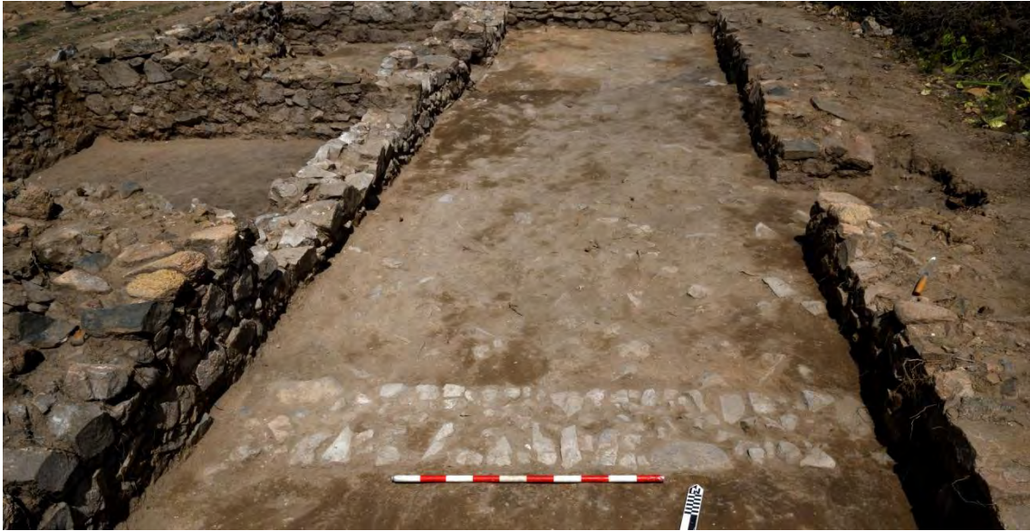
Final view of Space 3D3 from the south, with the partition wall between 3D2 and 3D3 to the south and the access door to the building to the east
