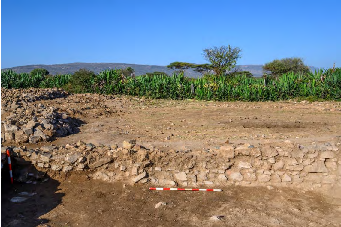
Detail of the SW corner of Room 3C, where two different construction techniques can be appreciated, the one to the left corresponding to a remodeling of the building
