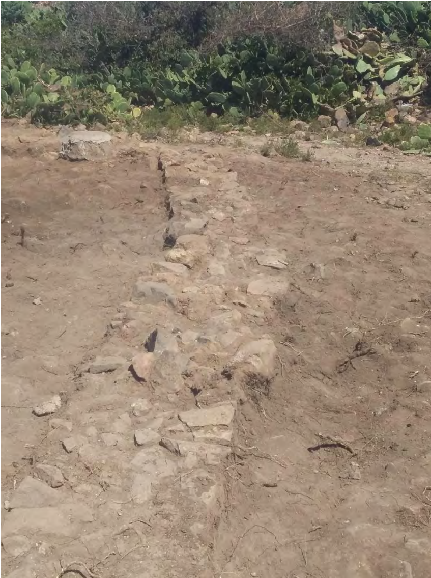
View of the southern wall of C-300, where a reordering of the direction following a remodeling of the building can be seen
