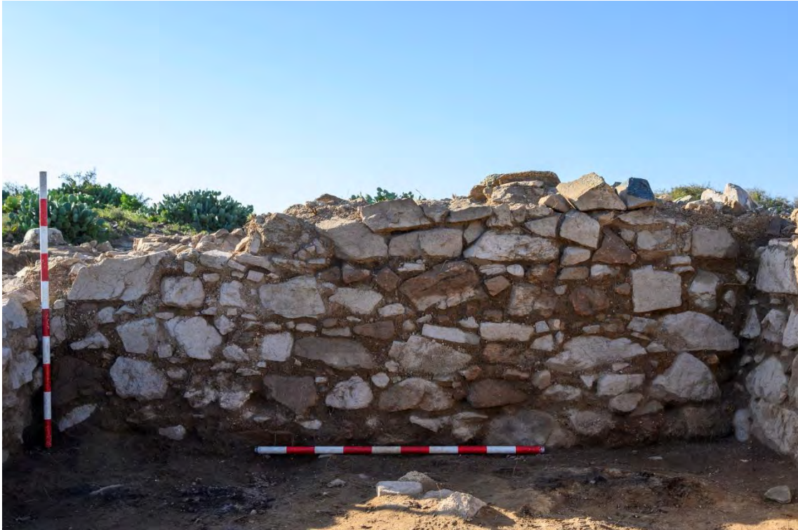
Southern wall of Room 3A, where the maximum height of C-3000 has been documented
