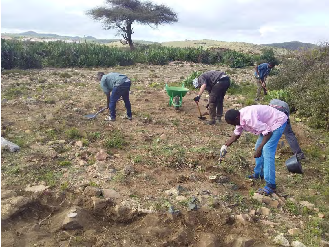
Clearing process of the excavation area
