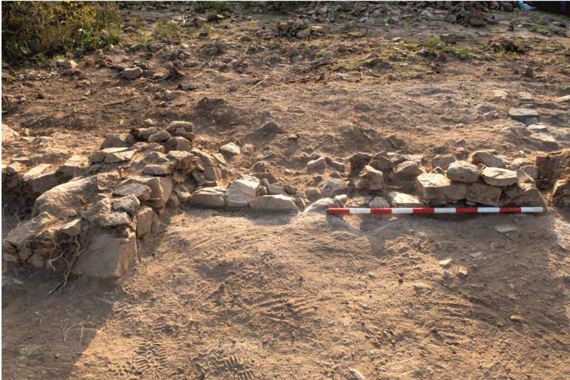
View of the damaged western wall of Room 4B from the east. To the left the partition wall with 4C can be seen
