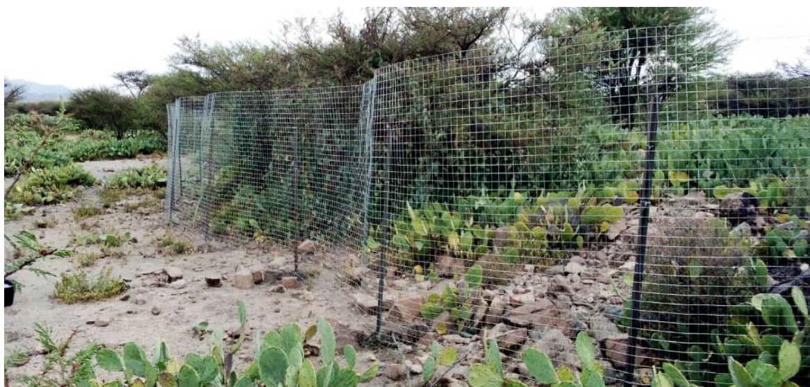
Construction of fencing at Abbasa site
